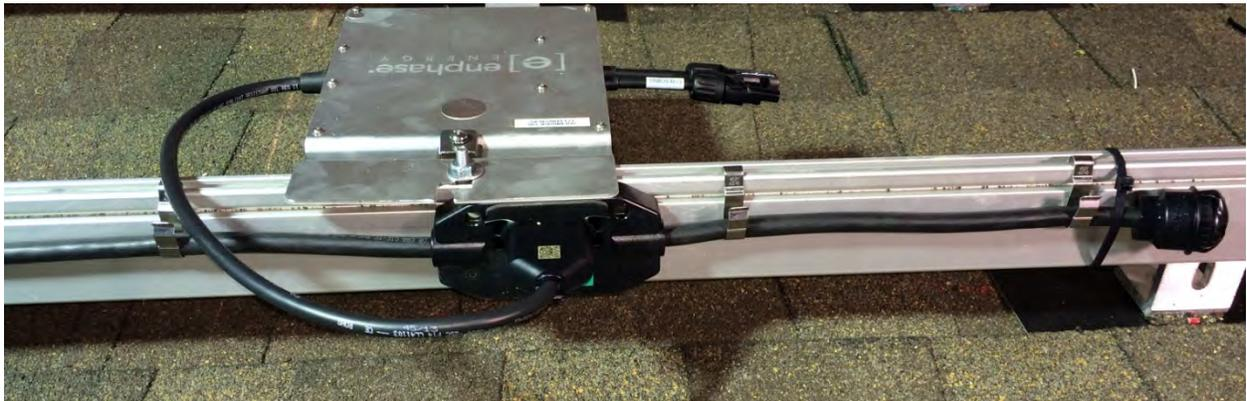
Install watertight seals (Enphase order: ET-SEAL) on all unused connectors on the Engage Cable to prevent water ingress into the cable, damage to the system, and potential fault conditions. Using these seals helps to eliminate avoidable service calls.
